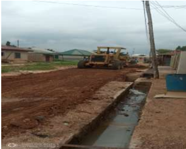
Plate 4: Road Being Graded by ECWA Church Source: Field Survey (2020)
