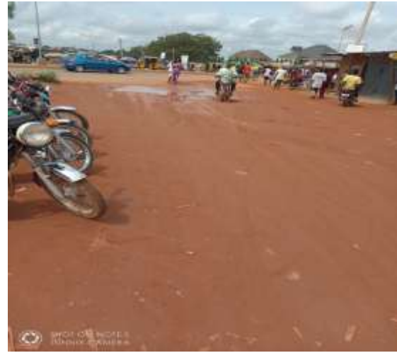
Plate 5: Earth Road Constructed and linked to Yakowa Way by Kamazo Community Source: Field Survey (2020)
