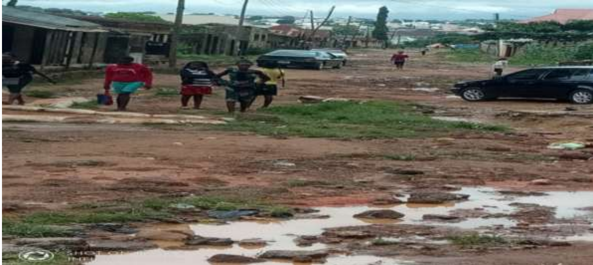
Plate 1: ECWA Hausa Road Unguwan Boro, vehicles meandering their ways on the bad road. Source: Field Survey (2019)
